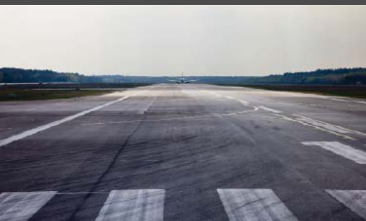
Runway Construction & Rehabilitation
